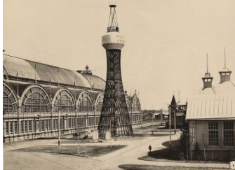
Shukhov Tower, a lattice 37-meter water tower by Vladimir Shukhov All-Russian Exposition, Nizhny Novgorod, Russia, 1896
